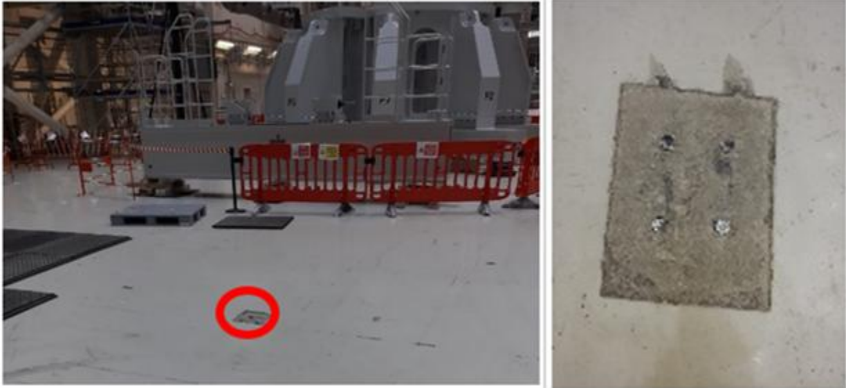
Figure 9-19: area in B13 slab with existing post-drill anchor cut flush to the slab
